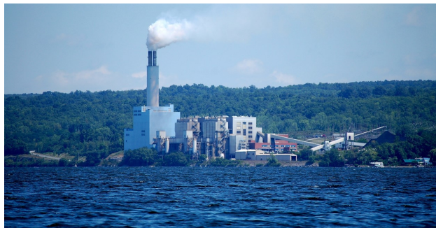
AES' Cayuga plant
